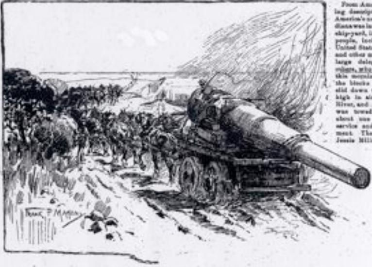
The New 23-ton Coastal Defence Gun. On the way to its site at Ben Buckler, near Bondi. The gun has a range of 12 miles, and throws a projectile weighing 600 lbs.
